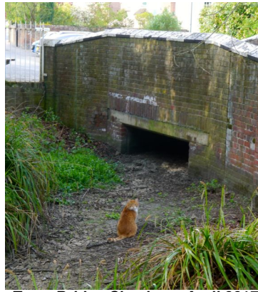
Town Bridge Chesham, April 2017
